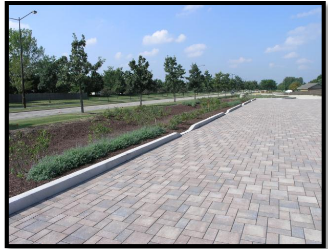
Above: Spring Lake Park, a Fox Valley Park District permeable pavement parking lot located in Aurora, Illinois.
